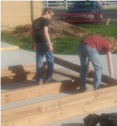
Nailing Rim Joist (Header) into place
